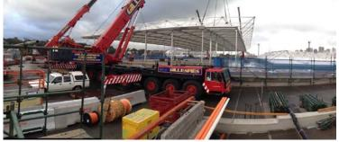
**ABOVE:** Four massive cranes swung into action earlier this week at the new Sydney Exhibition Centre @ Glebe Island, lifting the 150 tonne roof and frame for the largest of the exhibition halls into place.
