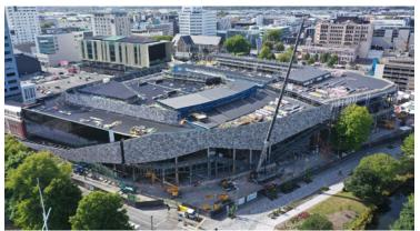
TE PAE Christchurch Convention Centre, pictured, has inched closer to completion ahead of its opening in Oct, with CPB Contractors having now installed a quarter of the 43.000 herringbone tiles that will form the braided river effect of the building's facade.
